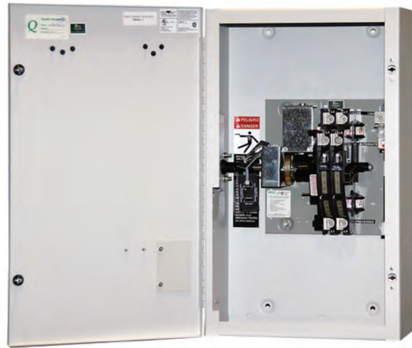
185 Manual Transfer Switch Door Open
